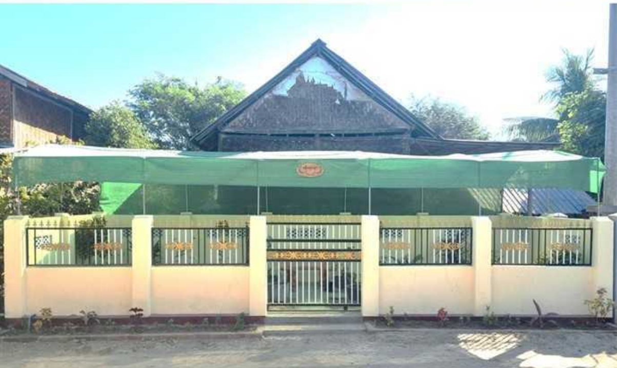
Figure 72: Completing Public Toilet and Community Garden Construction in Mann Kyoe Village
