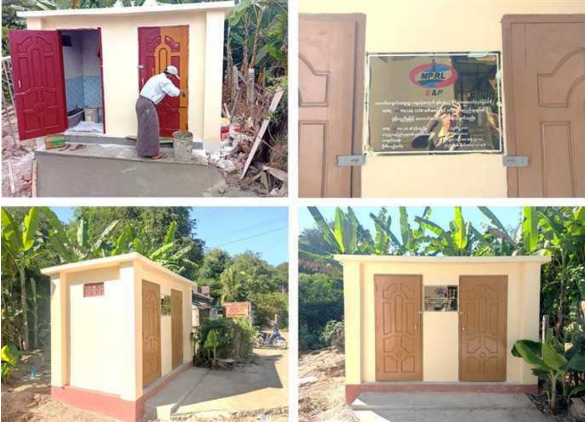
Figure 69: Completing Twin-pit Toilet Construction at Auk Kyaung Dhamayone
