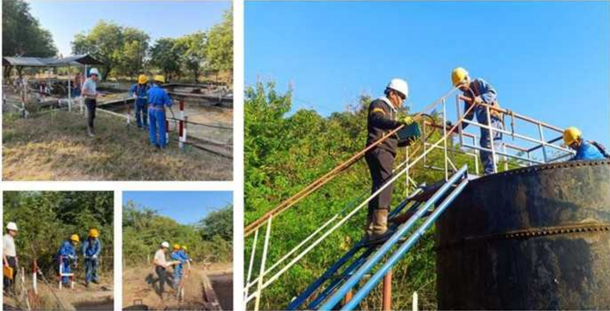
Figure 56: Tank walkway, Pit Safety Barriers Inspection and Maintenance
