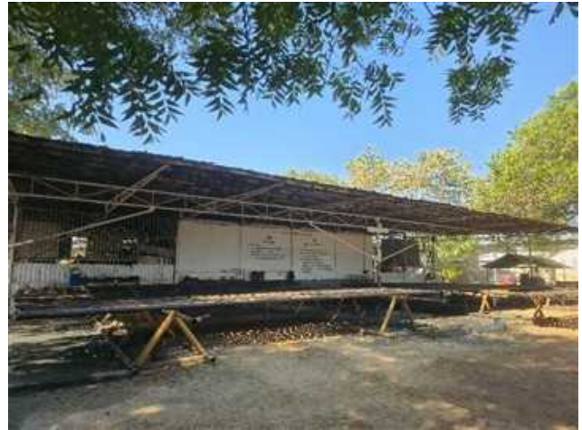
Figure 43: Warehouse Tubular Section
