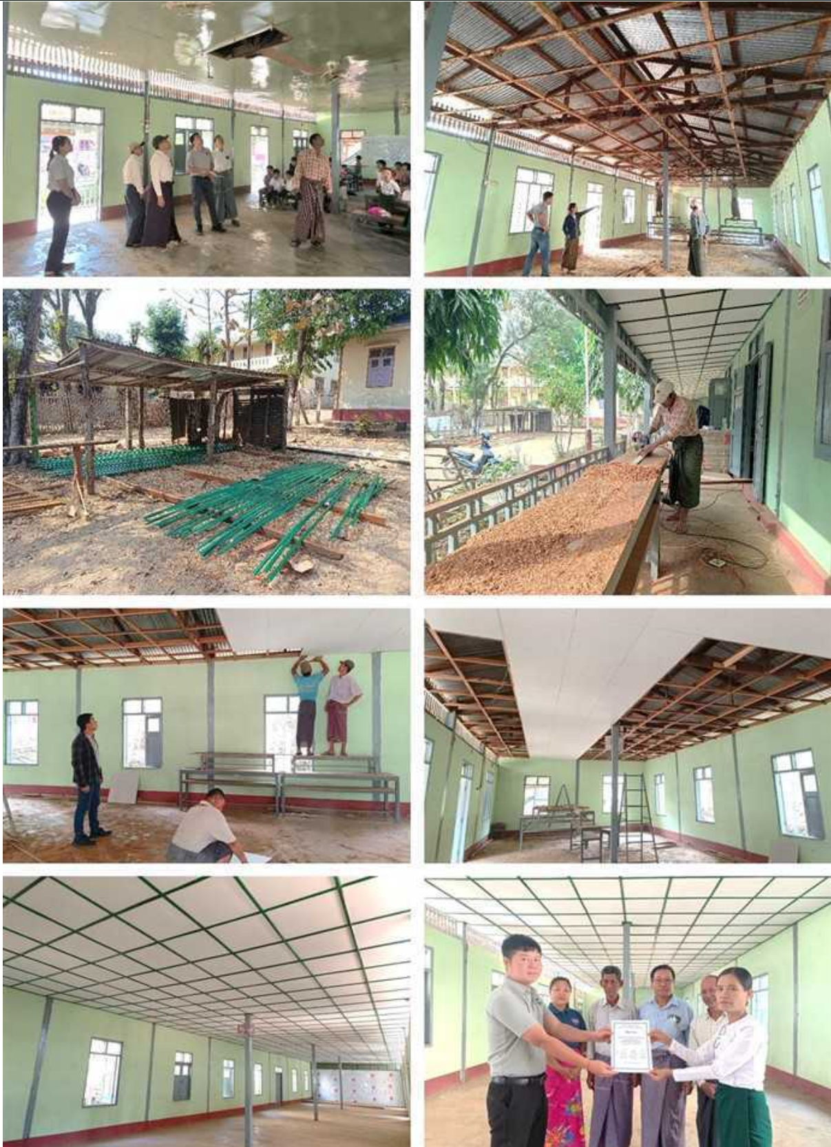
Figure 78: Completing Ceiling Installation at Lay Eain Tan Basic Education Middle School
