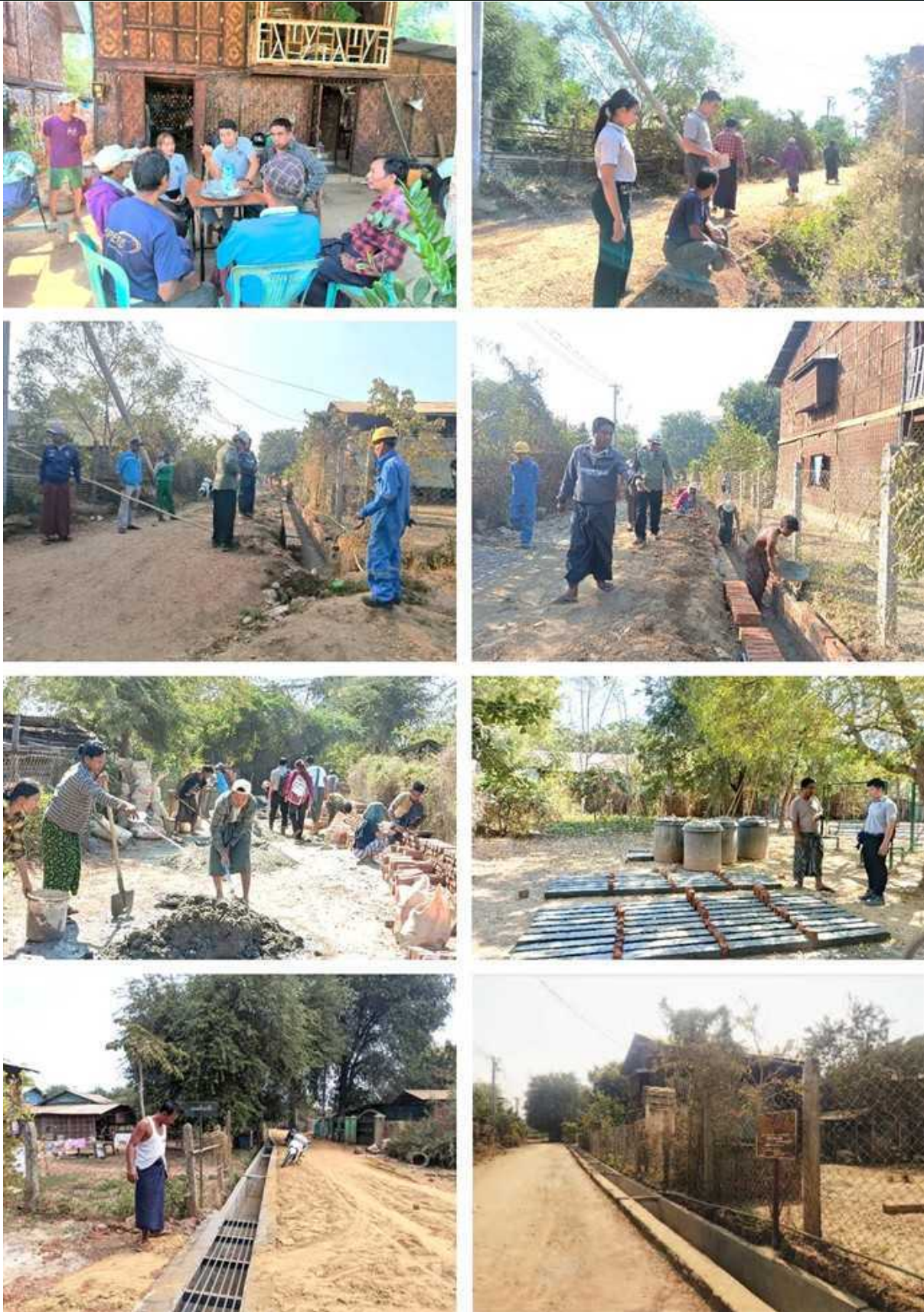
Figure 77: Completing Concrete Drainage System near Ma Kye Chaung School
