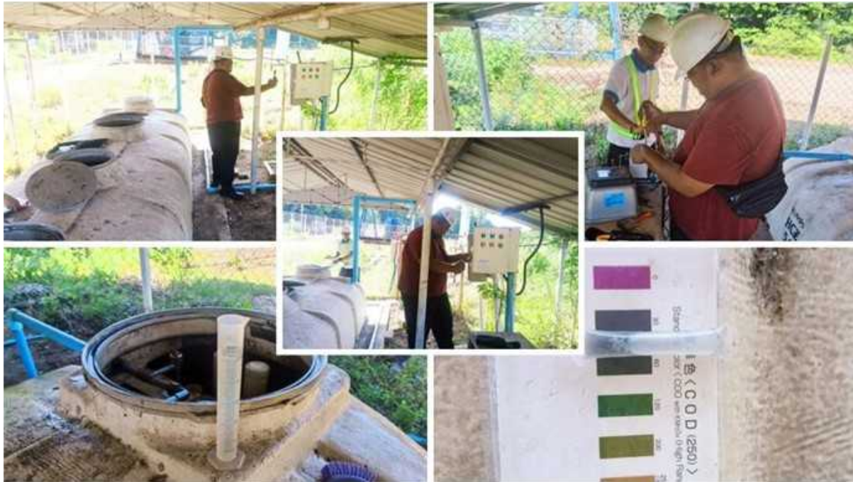
Figure 60: Contractor Inspection & Maintenance for Biofiltration Unit at Base Camp
