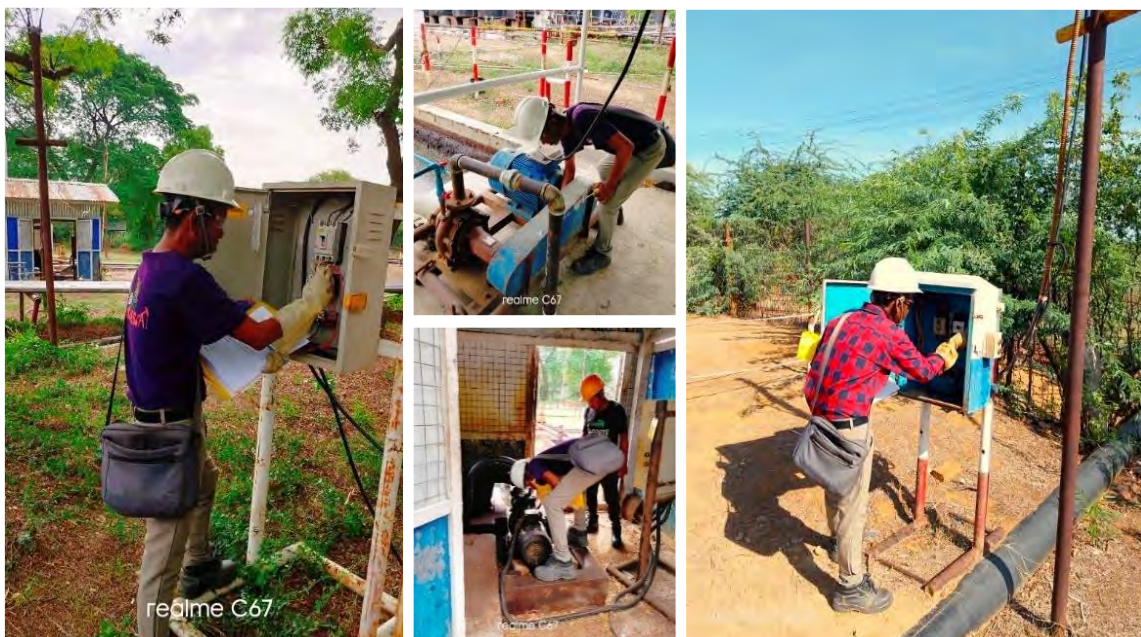
Figure 52: Electrical Equipment Inspections
