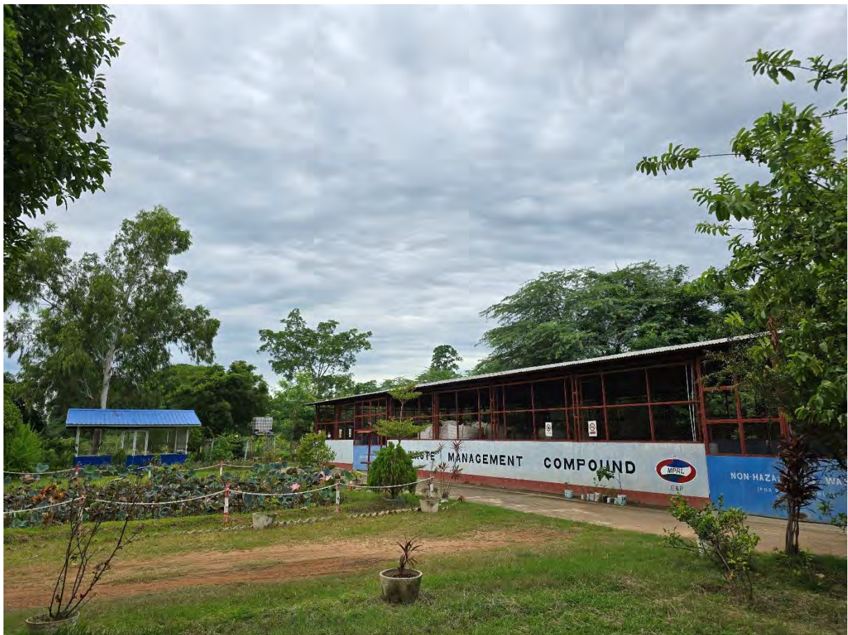
Figure 6: Waste Management Compound
