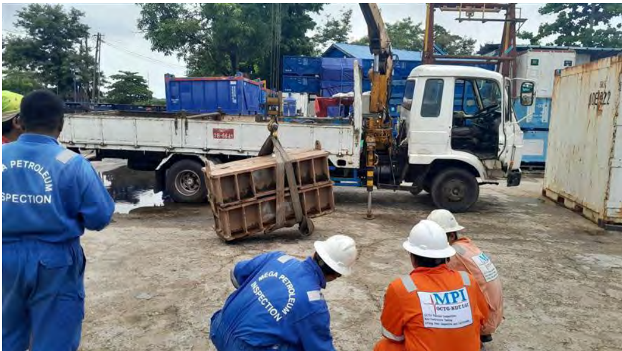
Figure 16: Contractor Inspections & Load test
