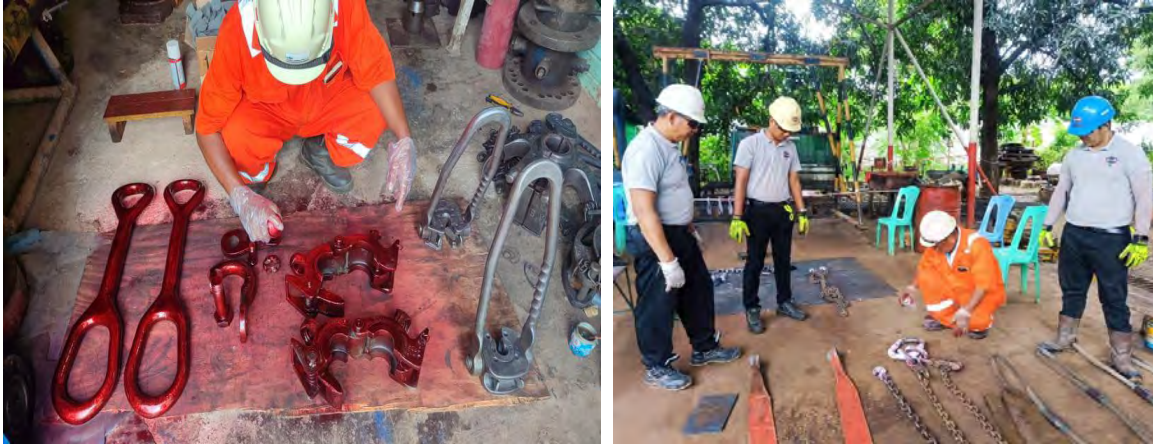
Figure 55: Lifting Gear, Hoisting & Handling Equipment NDT Inspection and Color Coding
