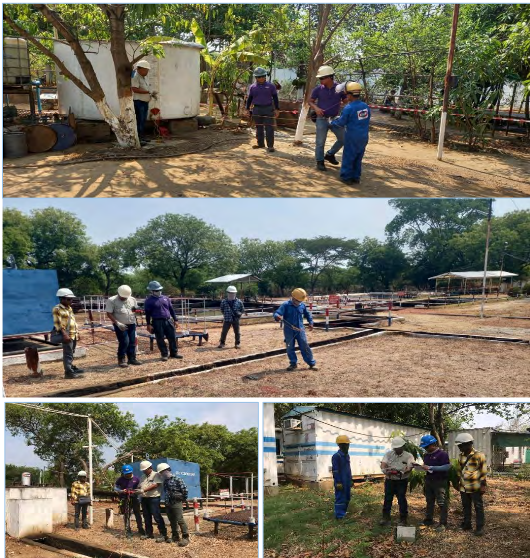
Figure 50: Earthing Resistance Test
