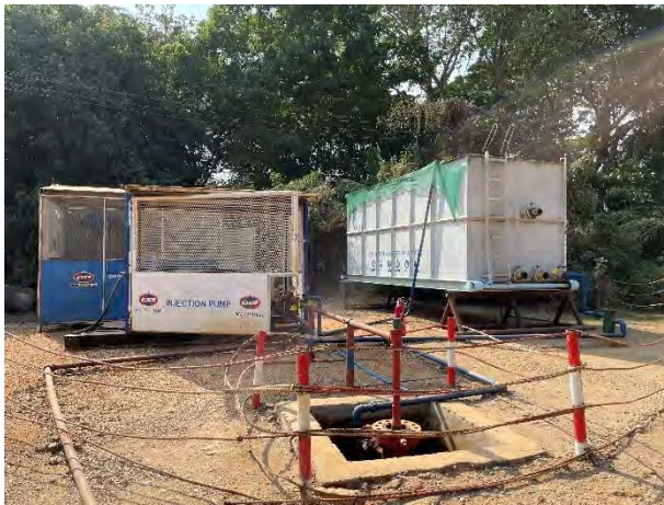
Figure 36: Produced Water Injection into Shut-in Wells
