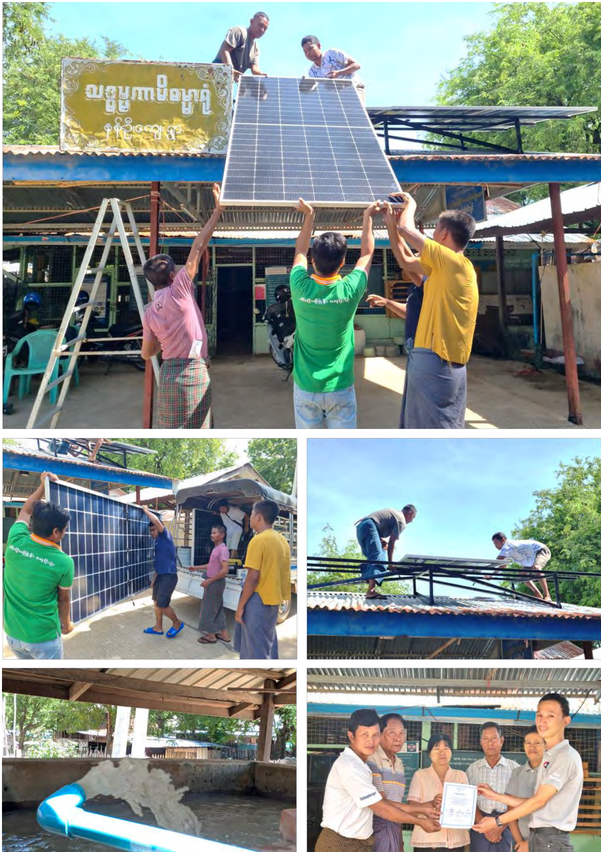
Figure 78: Transferring Solar-Powered Water Pumping Project to Nan U Village Development Committee
