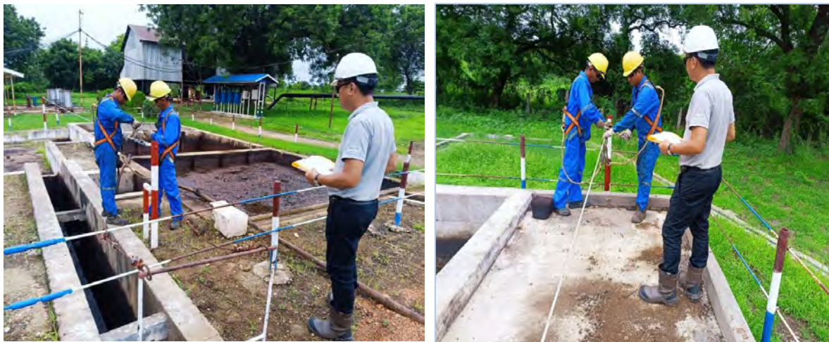
Figure 56: Inspection and Maintenance of the Safety Barriers
