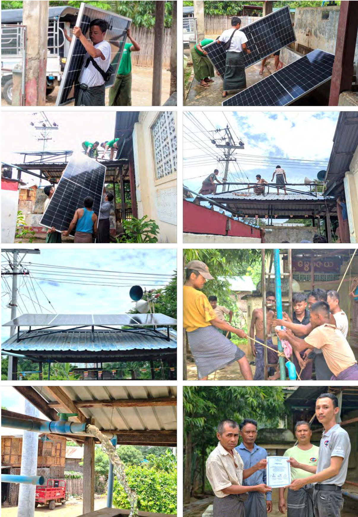
Figure 76: Transferring Solar-Powered Water Pumping Project to Pauk Kone Village Development Committee
