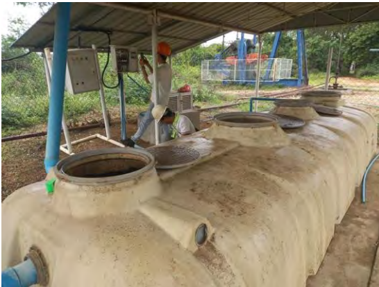
Figure 39: Regular Maintenance of Bio-filter by Third-party
