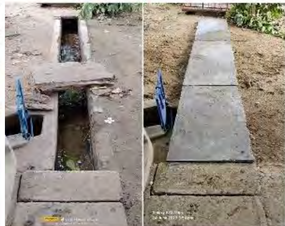
Concrete work for drain ditch covers. (STF-hazards findings)
