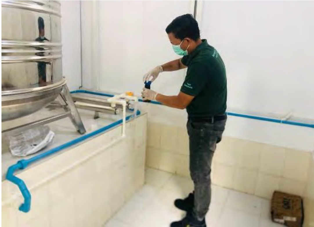
Figure 52: Water Sample Collection at RO Drinking Water System at Mann Field Base Camp
