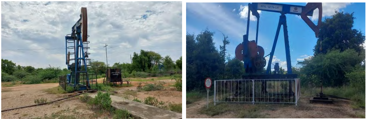
Figure 25: Concrete Pad and Additional Cellar at M-290 and M-554
