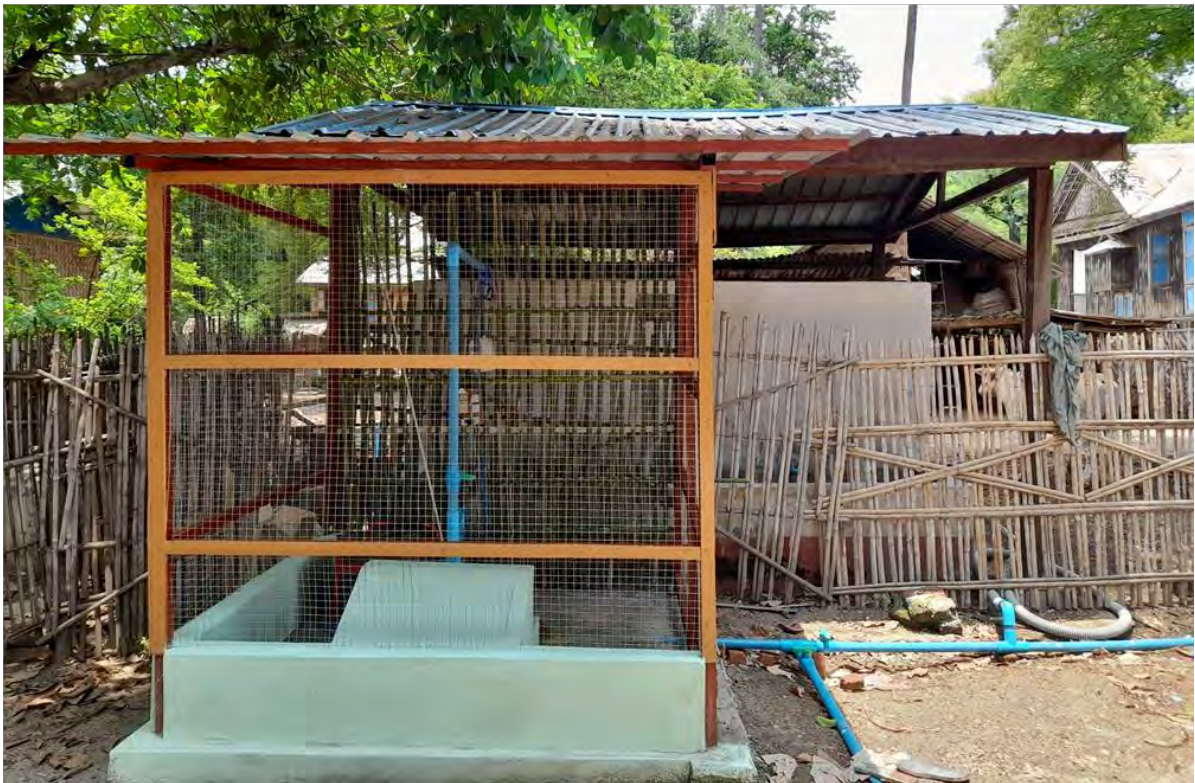
Figure 93: Completing Water Pumping Project in Chin Taung Village
