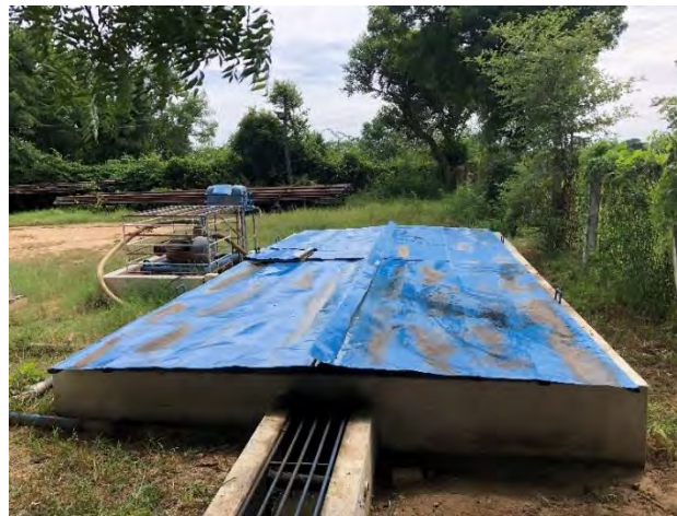
Figure 49: Warehouse Zero Discharge Tank
