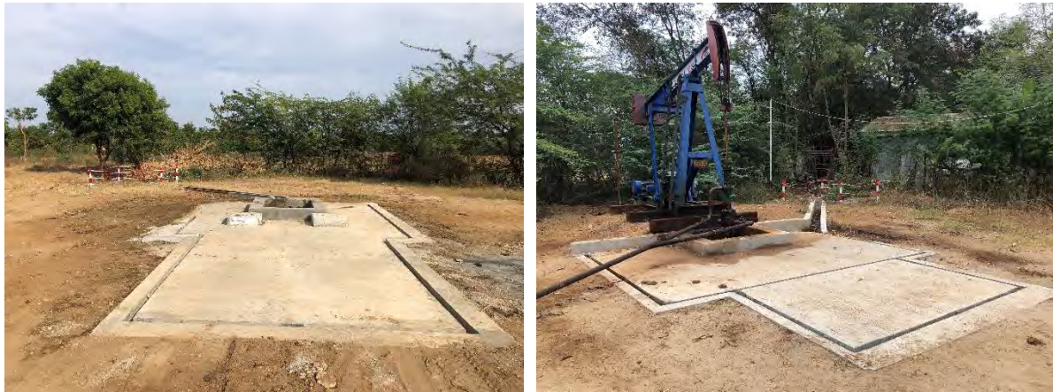
Figure 24: Concrete Pad and Additional Cellar at M-290 and M-554
