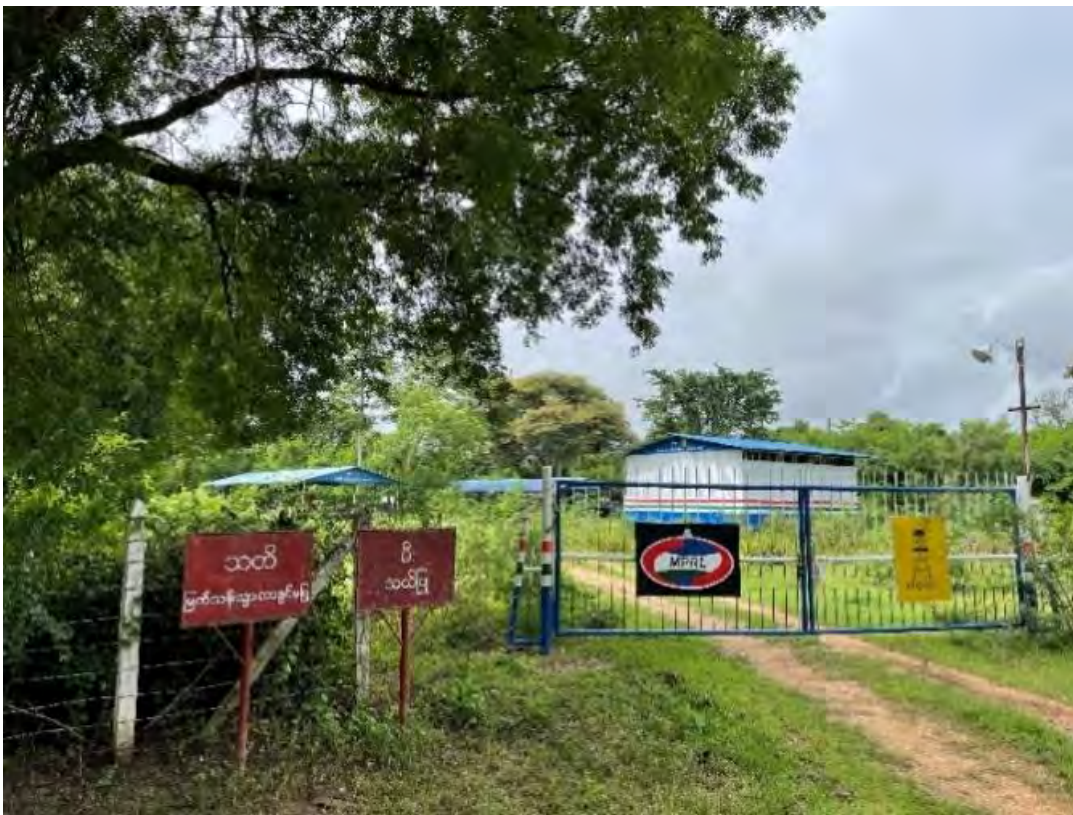
Figure 43: Sludge Management Compound (SMC)
